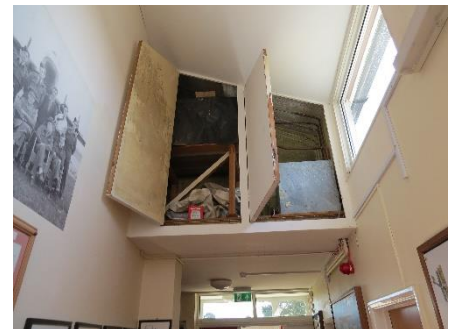
Hall Lobby showing redundant ceiling cupboard and water tank
